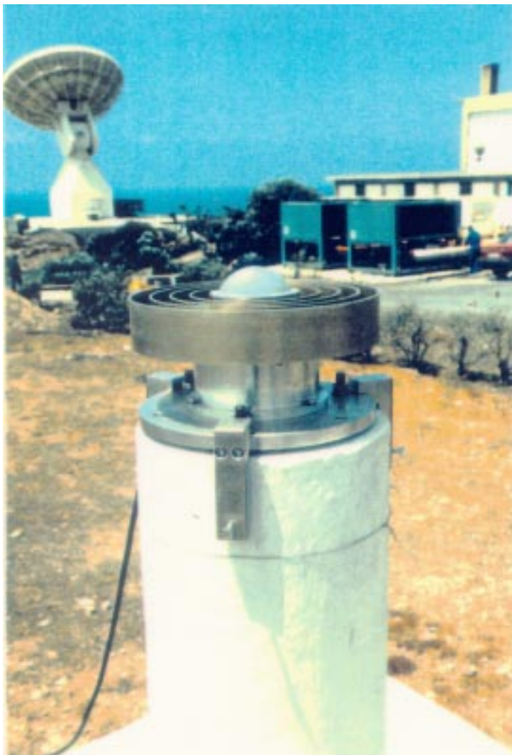
Figure 4. GPS antenna and pillar in Maspalomas, Spain.
